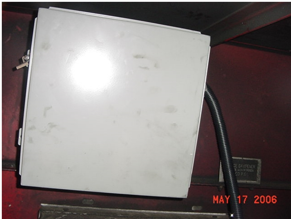
De-Icer's mount the ECM in weatherproof enclosure inside of rear compartment.
